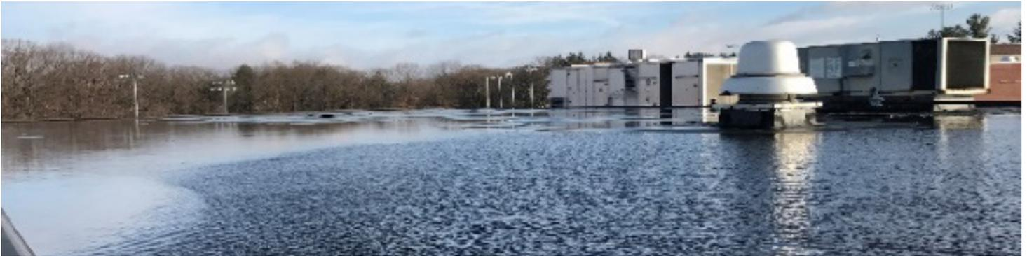
**Water remained on the roof, creating several inches of standing water (or ice), as well as leaks within the building.**
